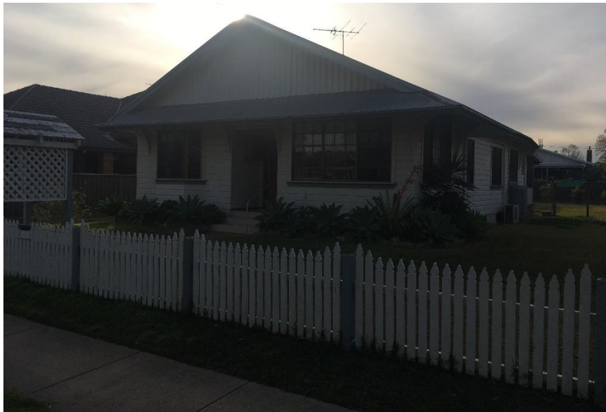
Figure 3 – Existing house on site to be demolished
