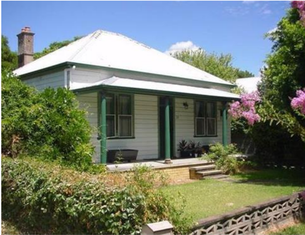
29 Allan St – Before Rear additions
