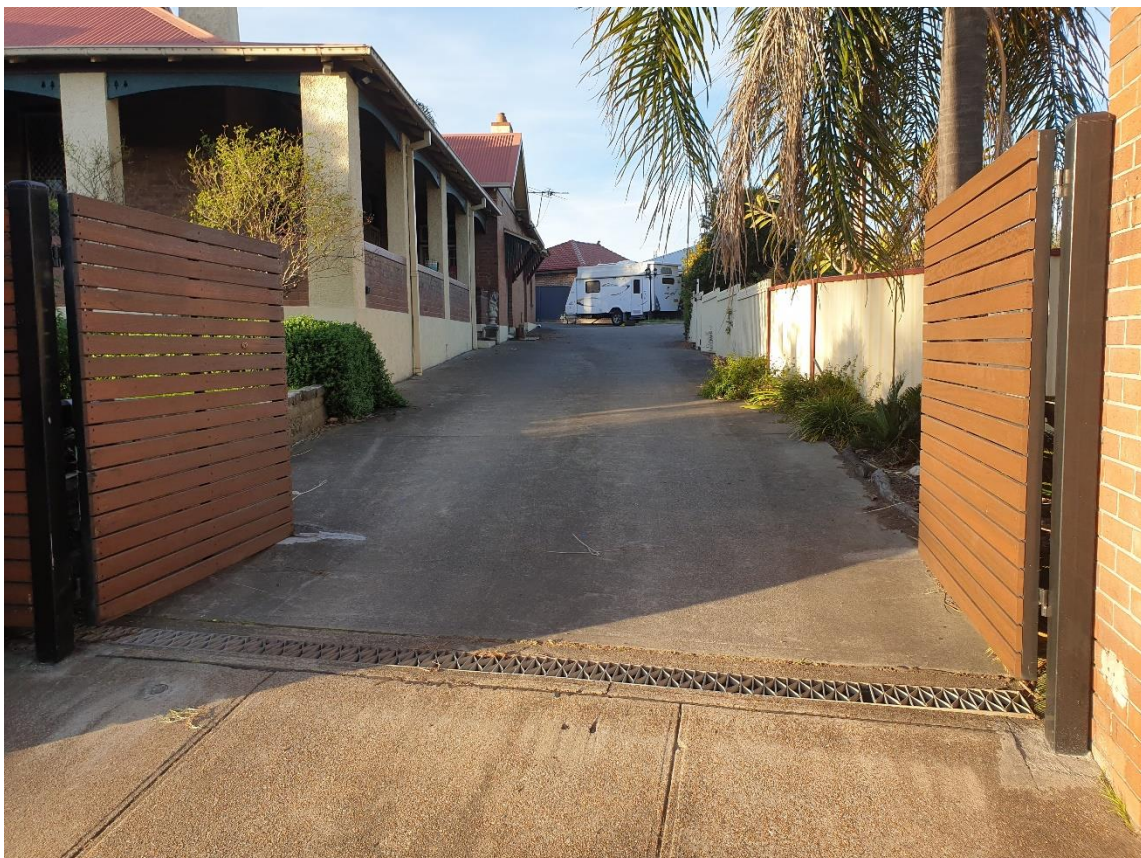
Figure 7: Photo of Existing Driveway & Gates (June 2021)
