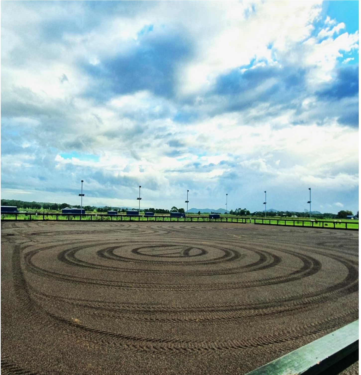
Figure 10 – February, 2022 Final Arena Completion with full compliance with works completed by Professional, Mr Greg MEXON, Mexon Earthworks.
