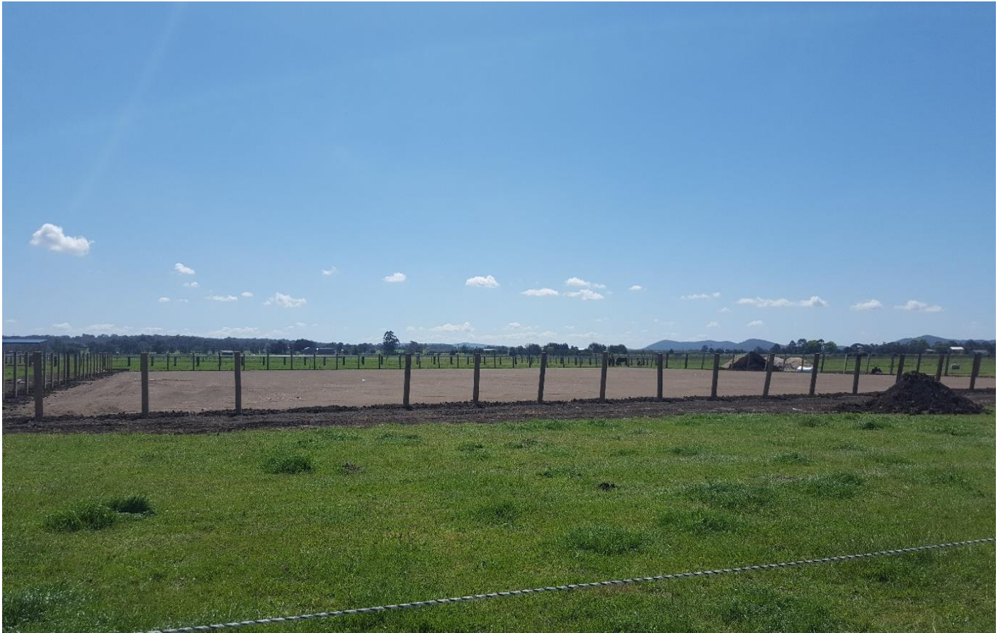
Figure 8 – 2018 Commencement of arena minor excavation.
