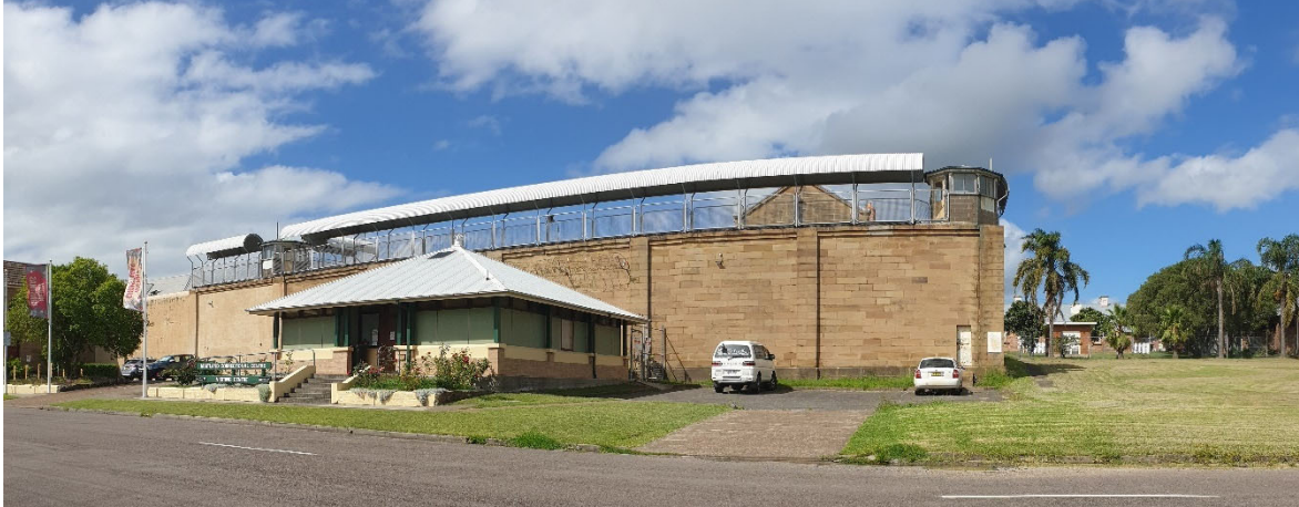
South-west facing prison wall of Maitland Gaol - Tower 6 at right and Tower 1 at left (sheltered gantry walkways in between)
