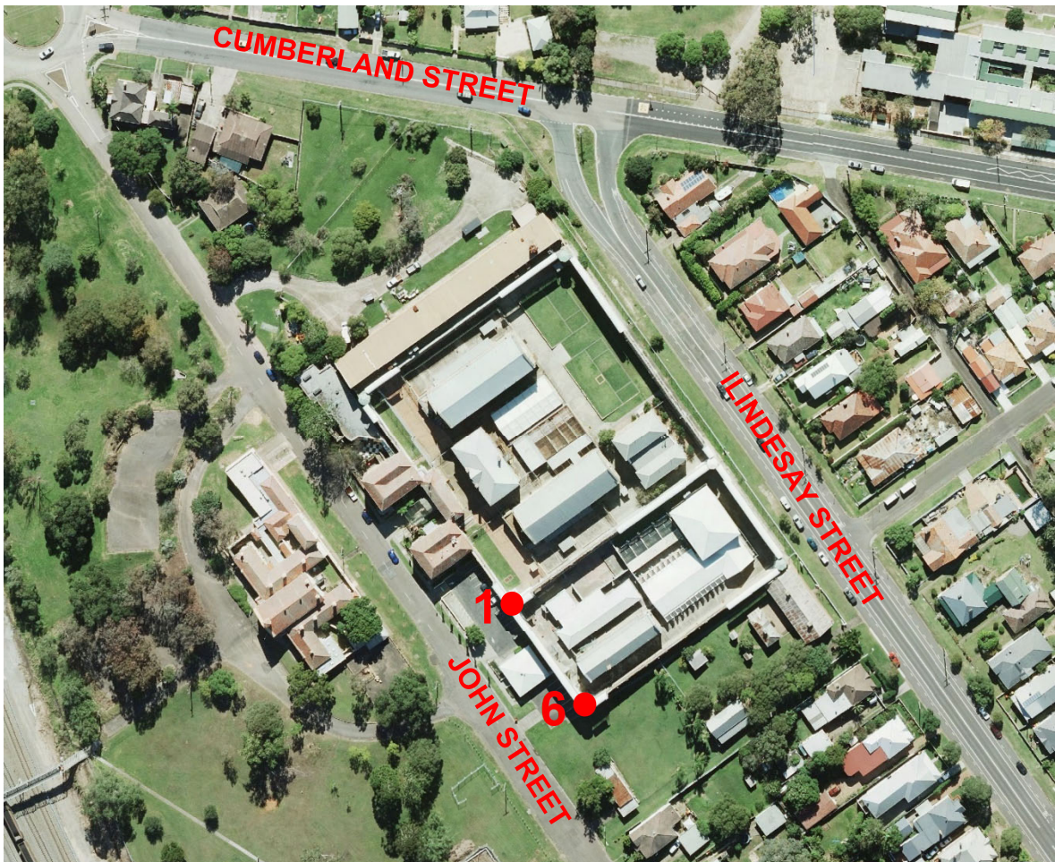
Aerial Photograph of Maitland Gaol with Towers 1 and 6 marked red (Image source: NSW Govt. SixMaps)
