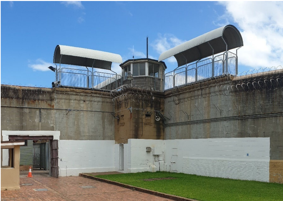
Tower 1 viewed from within former prison yard looking south – Gantry Walkways 1 and 2 in foreground
