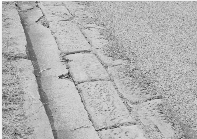
Example of bitumen extending over the sandstone kerb and guttering
