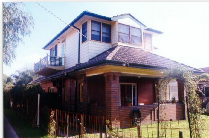
The second storey addition to this building overwhelms the original structure and destroys its identity
