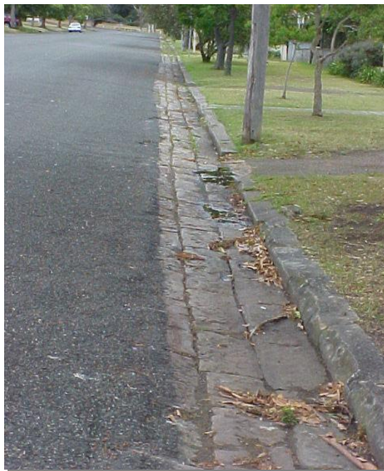
Sandstone Kerb and Guttering in High Street
