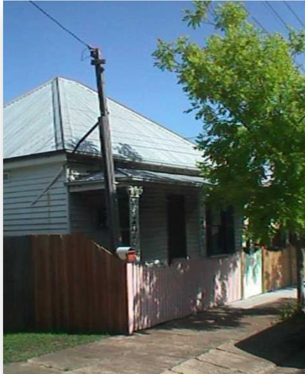
Alterations to this Victorian cottage returned the verandah to its original hipped form. A fence in keeping with the age of the building was also constructed
