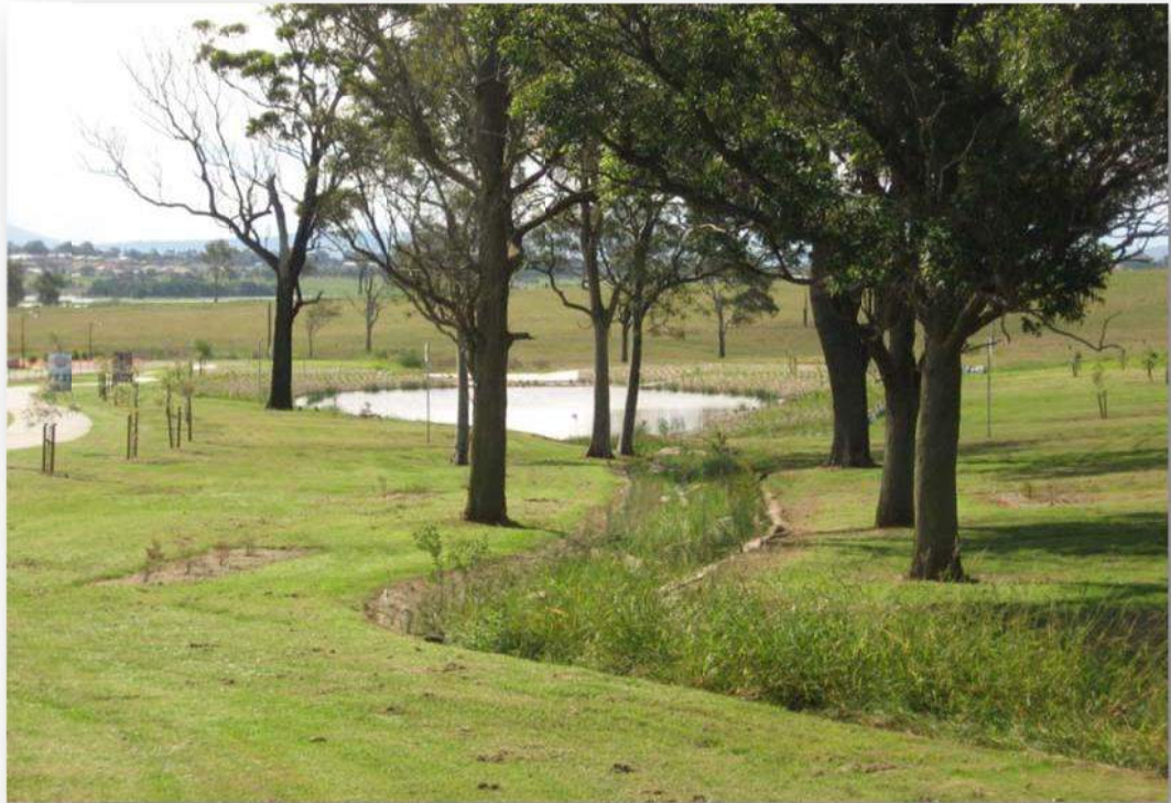
Figure 8: Urban drainage network identified in Figure 7 above, showing detention areas further downstream. These detention areas eventually link with flood prone land further North.
