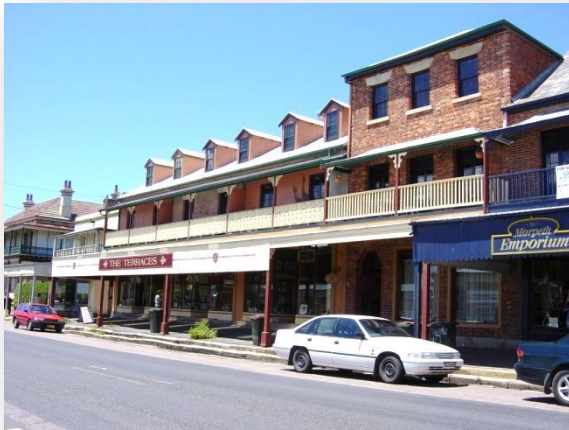
Verandahs across footpaths should be constructed only where documentary evidence exists as to their original design.
