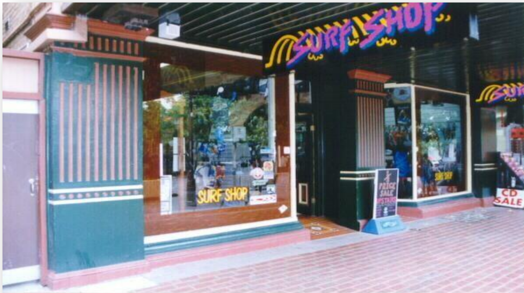
The restored shopfront to this shop in High Street attracts public attention and gives a feeling of quality to the shop
