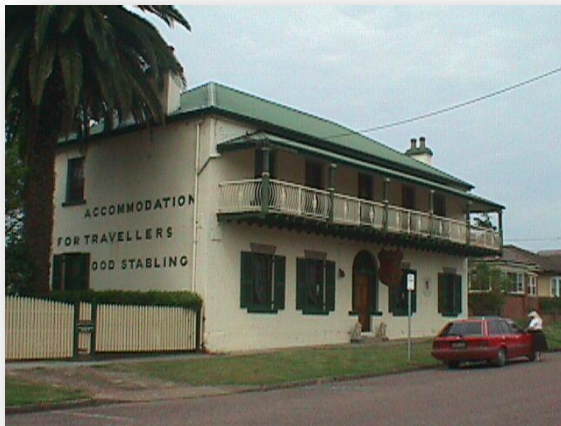
An early Georgian two storey building in East Maitland
