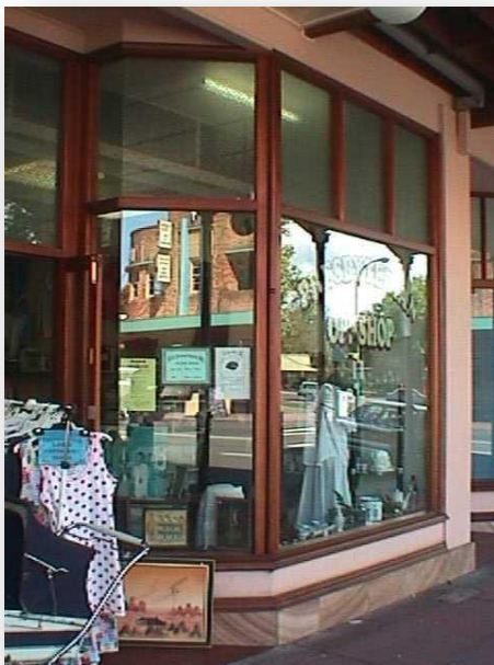
New shopfronts in the historic High Street Glebe Trustees buildings were reinstated based on historical photographs.
