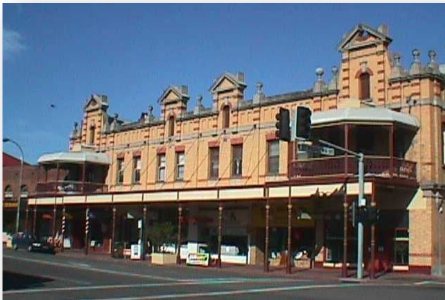
The verandahs on the Glebe Trust Building in High Street, Maitland were reconstructed using early photographs and plans of the original building
