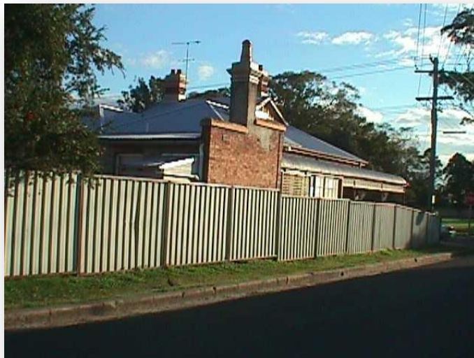
The colourbond fence used along the side boundary of this house detracts from the character of the building and street
