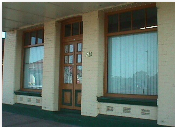
Early shop fronts are characterized by deep timber mouldings and the use of colour
