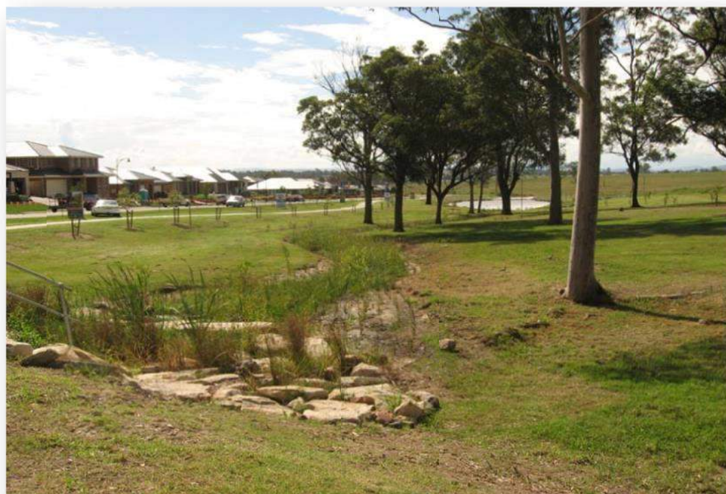
Figure 7: Urban drainage networks can be designed to assimilate with riparian land and waterways further downstream, as shown here at Chisholm. Note the proximity of the footpath to the riparian drainage network, which capitalises on amenity.
