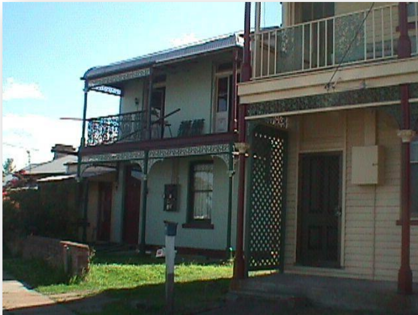
The original verandah balustrade and frieze of this building (left) had been removed, however, the owners are now carefully reinstating these features based on the original design
