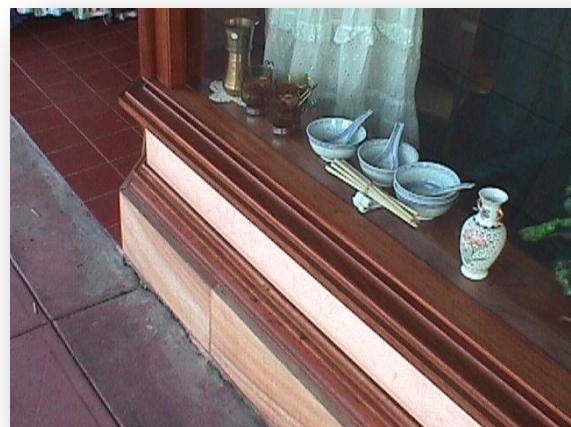
Deep timber mouldings characterise early shopfronts and are encouraged for new shopfronts where the original has been removed.
