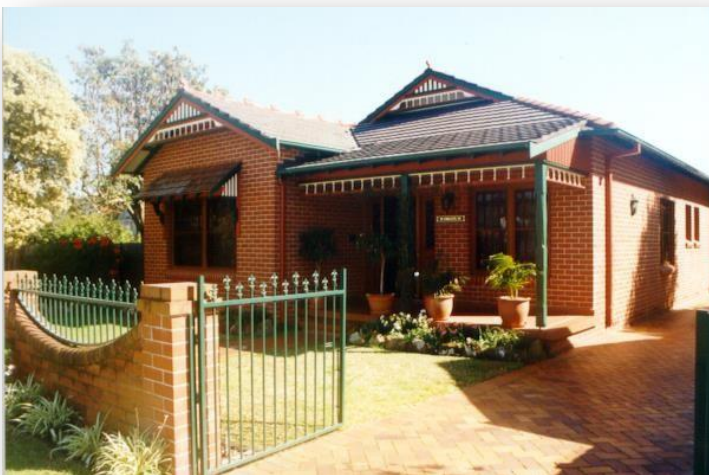
Architectural replicas or mock reproductions can confuse the old with the new, detracting from original buildings in a Conservation Area.
