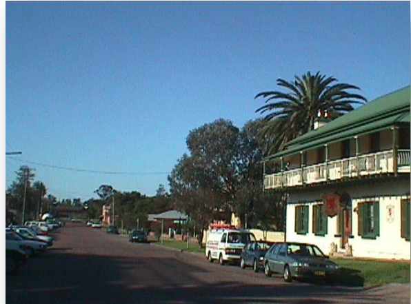
Banks Street defined the eastern edge of early commercial development in East Maitland
