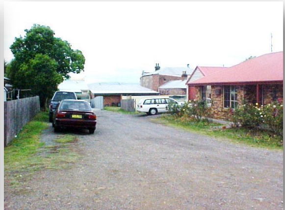
Land fronting Close Street at the rear of Swan Street commercial properties to be retained for service access and parking.
