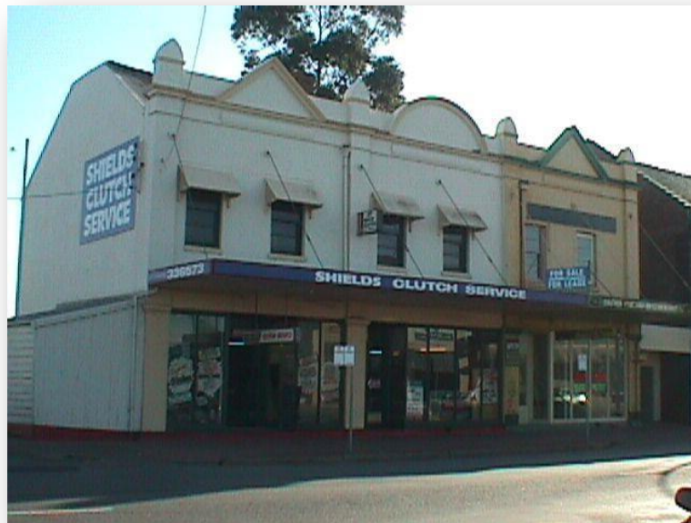
Original shop fronts add variety and richness to the streetscape and should be preserved
