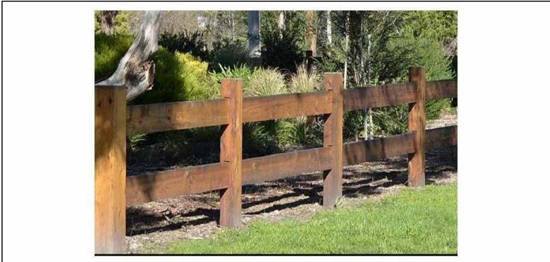
Figure 63: Typical Timber Boundary Fencing for Allotments Adjoining the New England Highway and Winders Lane.
