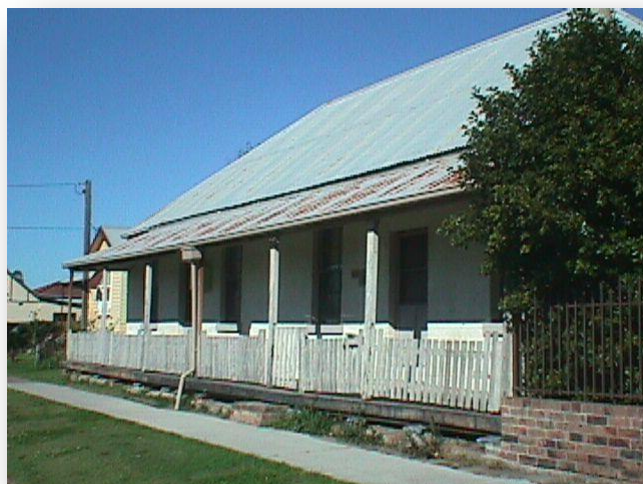
Some fences may be modest, but everyday fences contribute significantly to the character of the building and the area
