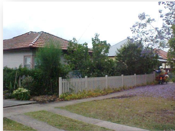
Simple picket fencing to a c1940's building
