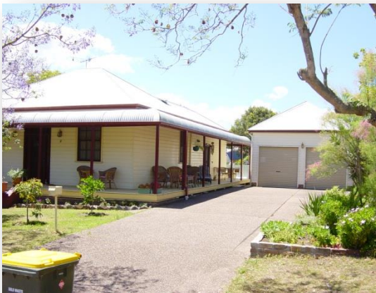
Double garage behind the rear building line of a residence
