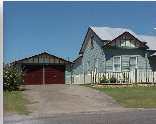
Double carports or garages should be located behind the main building line, and be constructed of materials consistent with the main house or in a timber weatherboard
