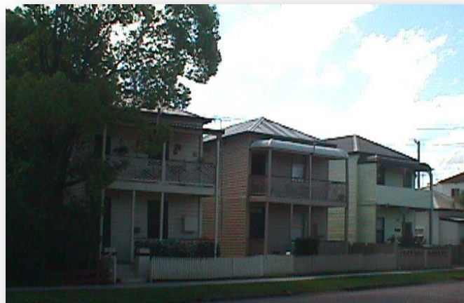
A group of single fronted houses in Anzac Street
