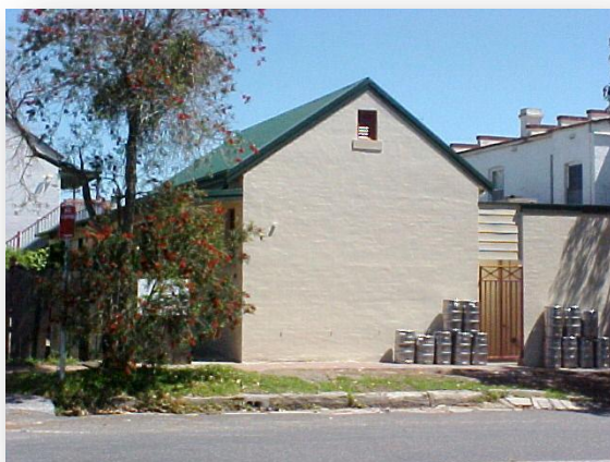
Sympathetic building forms and modern, but simple detailing have been used in this commercial development
