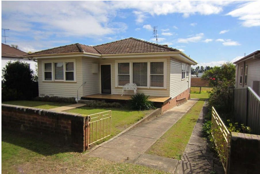
Existing dwelling to be demolished.
