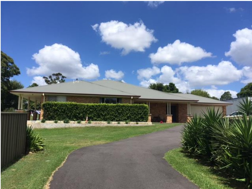
Figure 7 – Photo of existing dwelling at 23A Robert Street Tenambit – to be retained
