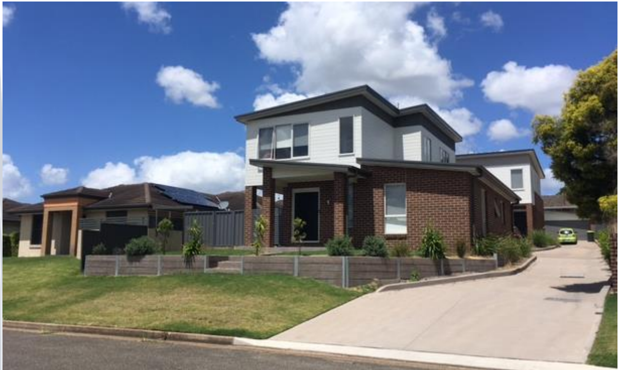
Figure 12 – Photo of recently constructed two storey units at Crawford Avenue Tenambit
