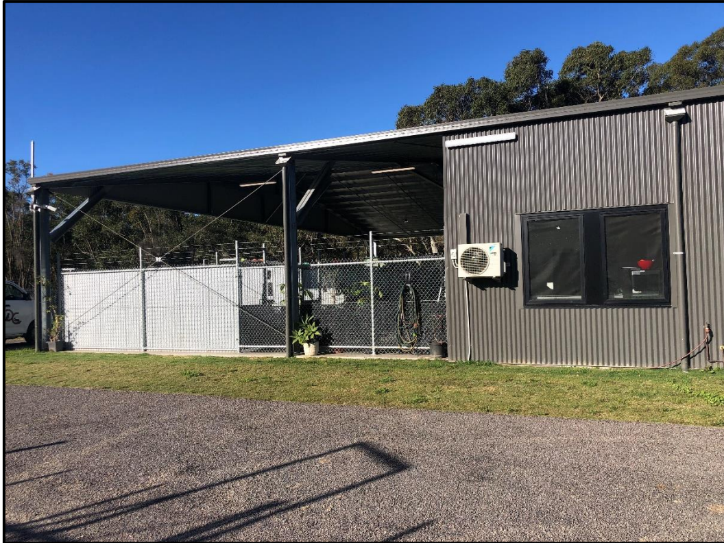
Photo 4: Side of existing Pound building on-site comprising kennels
