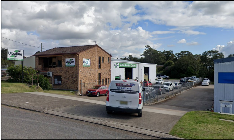
Figure 6: Agro Automotive located west of the site (view from Turton Street)
