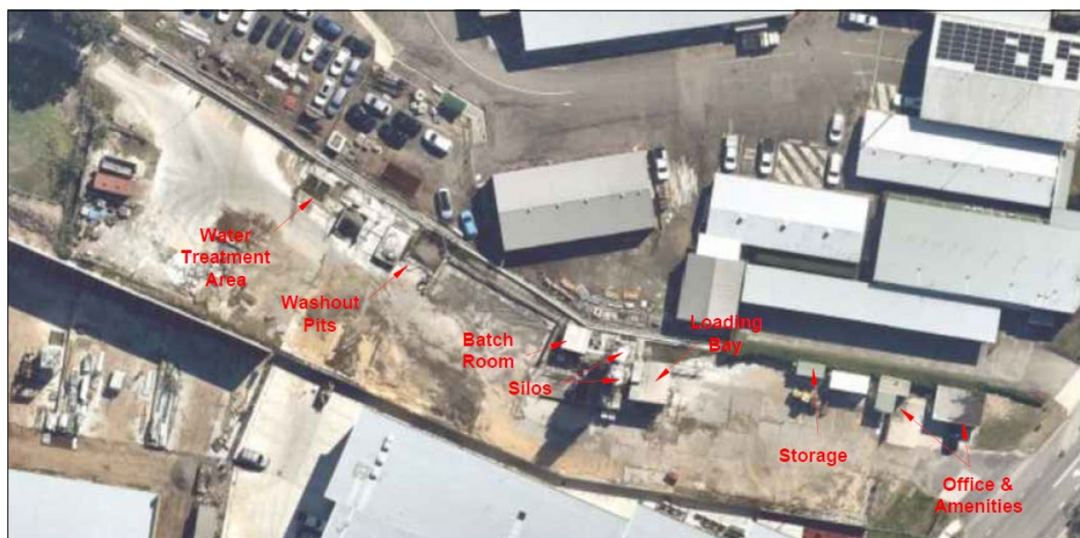
Figure 3: Existing buildings and structures on site
