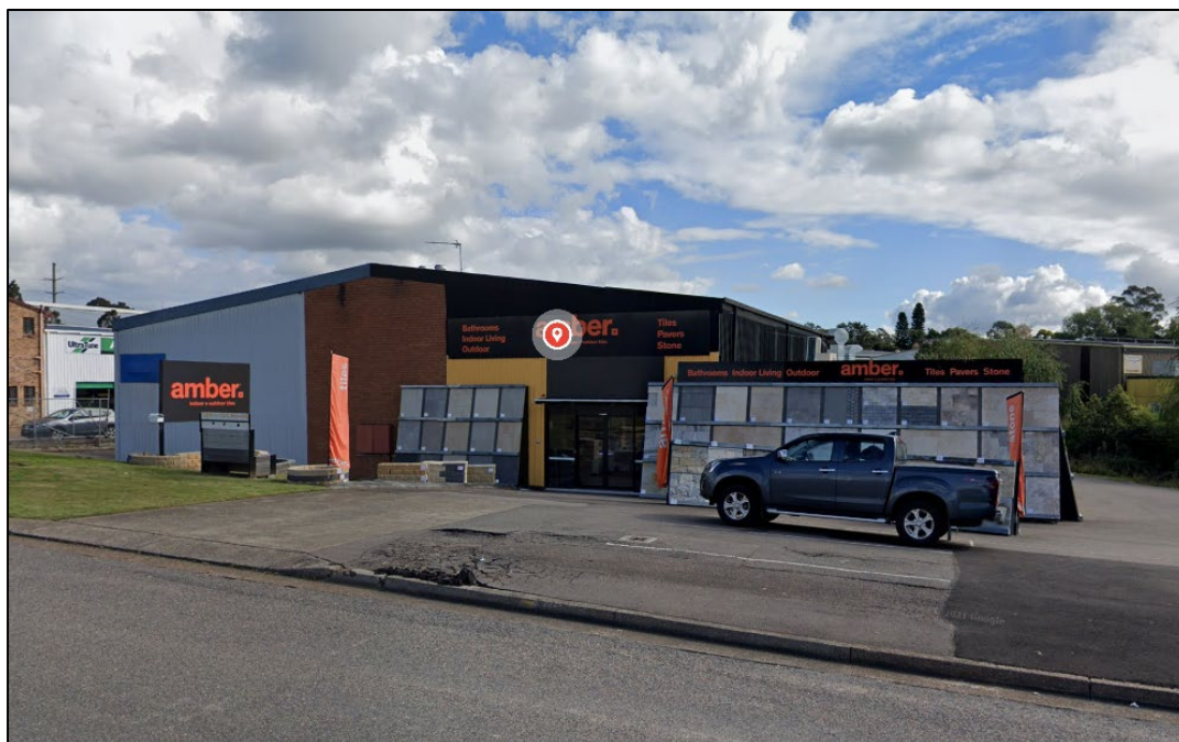
Figure 5: Amber Maitland located west of the site (view from Turton Street)
