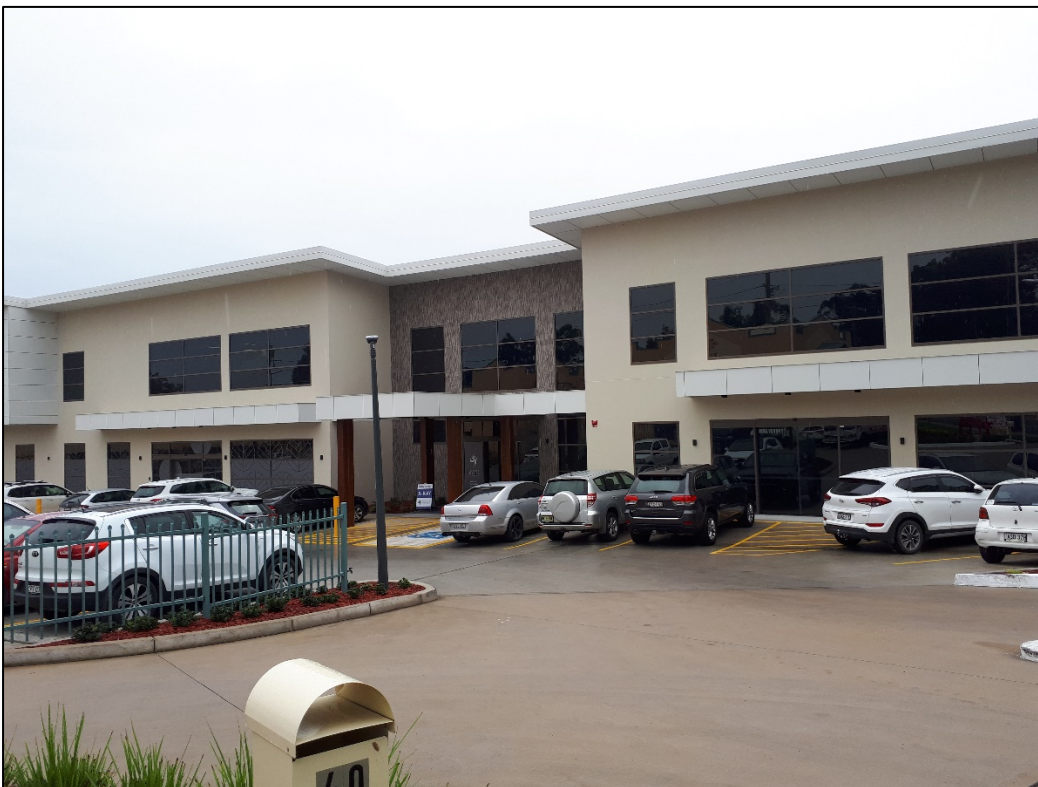
Figure 9: Hunter Imaging Group located south of the site (view from Metford Road)
