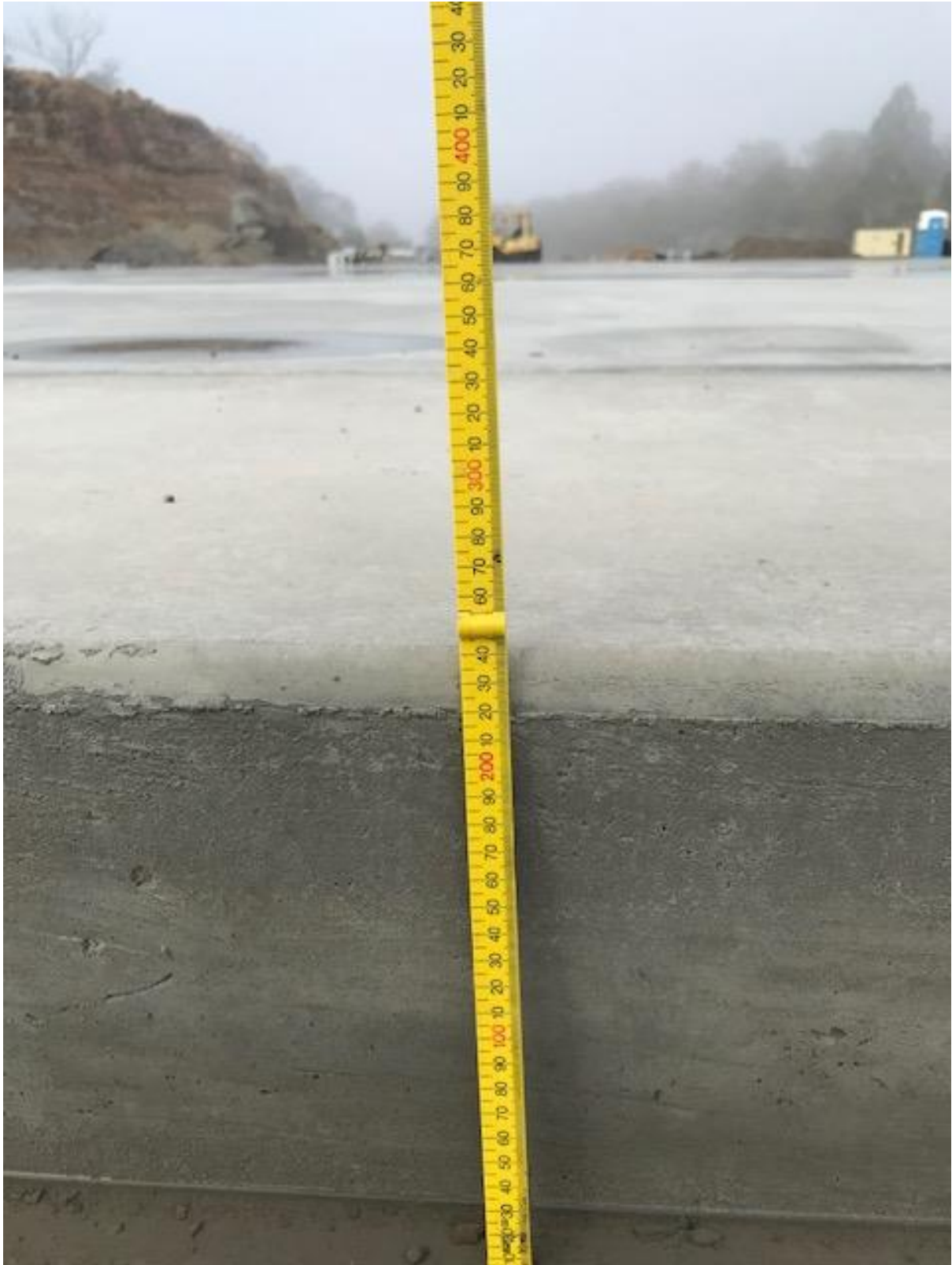
Figure C-2: In-situ concrete floor depth of shredder shed
