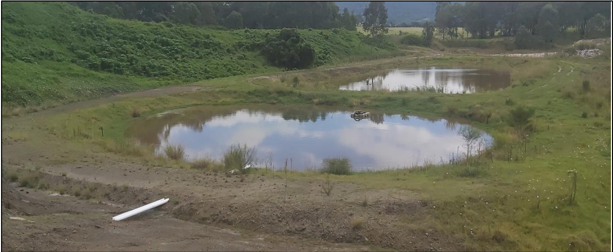
Above: Leachate Dams 1 and 2 operating levels in February 2022
