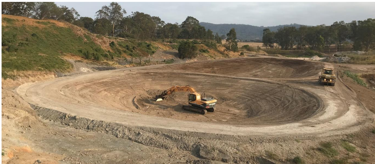
Figure 1 – Construction of Leachate Dam 1 (foreground) and Leachate Dam 2
