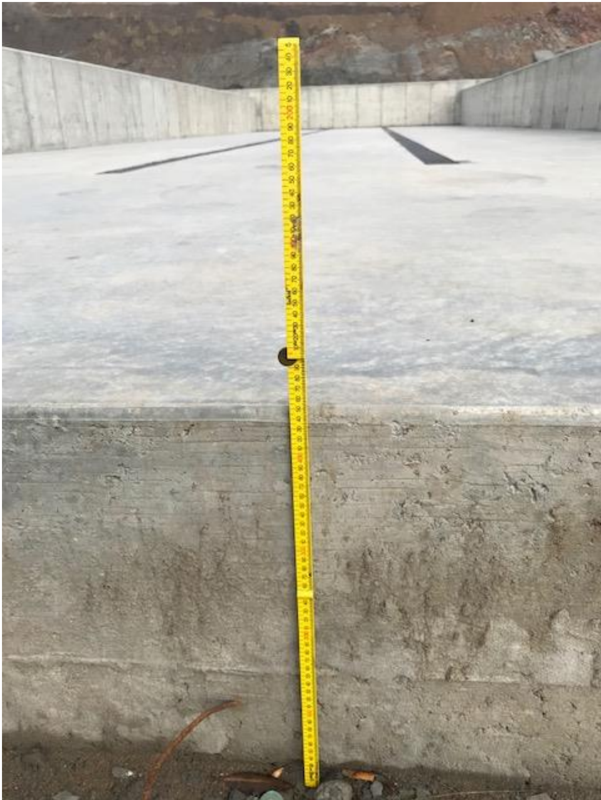
Figure C-1: In-situ concrete floor depth of composting bunkers
