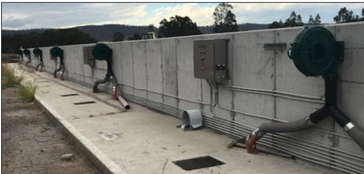
Above: Constructed concrete bunker with pair of dual purpose channels for aeration input and leachate drainage. Below: Air compressors mounted at the back wall of each compost bunker and covering plates over a pair of leachate drainage sumps per bunker.
