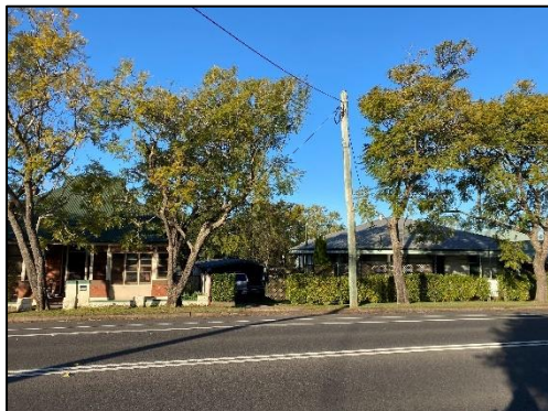
Photo 3: Front view looking south west
