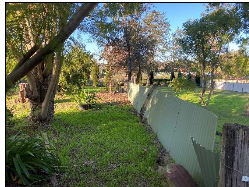
Photo 14: View along western side boundary, looking south
