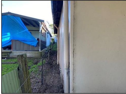
Photo 15: View along western side boundary, looking north
