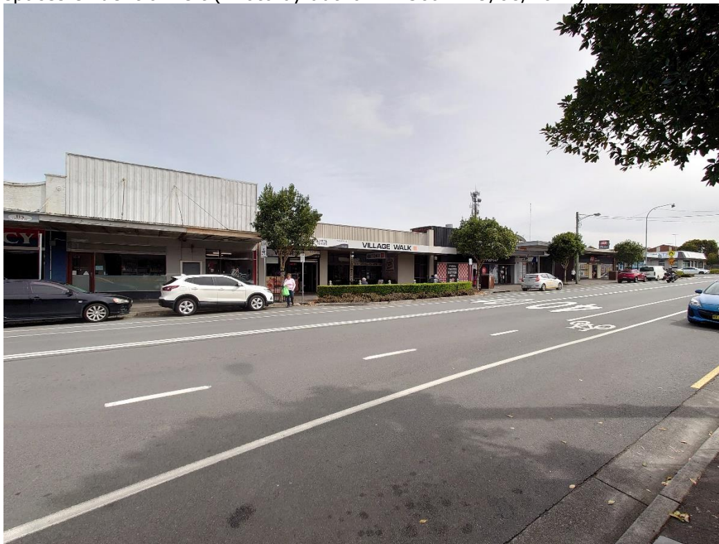
Photo 10: General streetscape view of Lawes Street opposite the site, note availability of on-street parking centre right (Photo by author August 2022)
