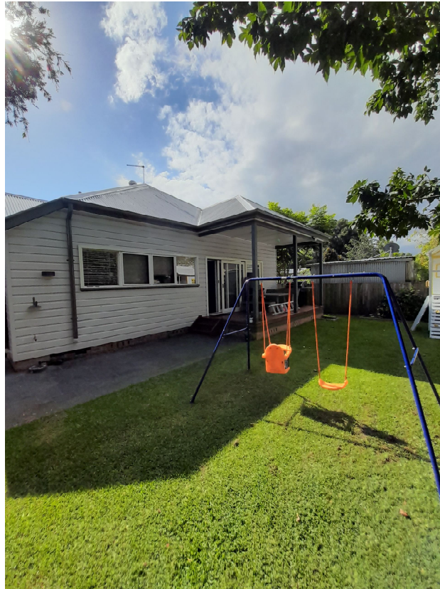
Figure 4 – Rear view of existing 16 Lorn Street
