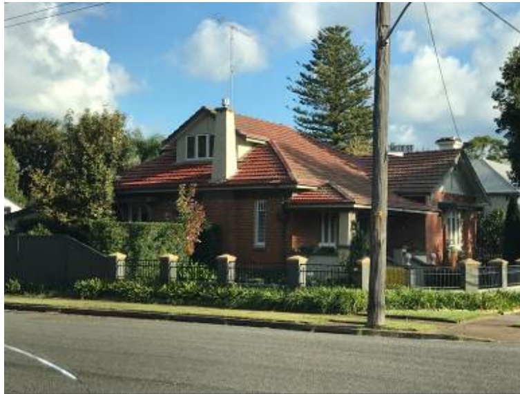
Dorma window addition to existing large bungalow roof Lorn – Gable and trims features
