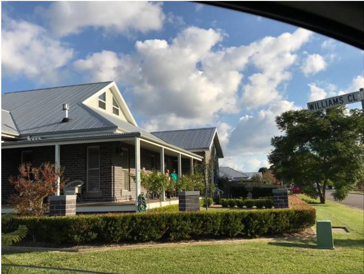
Corner of Williams Close and Melrose Street – Gable windows - not even traditional style but modern angular – colorbond fascia – colorbond gutters – contemporary dark brickwork
