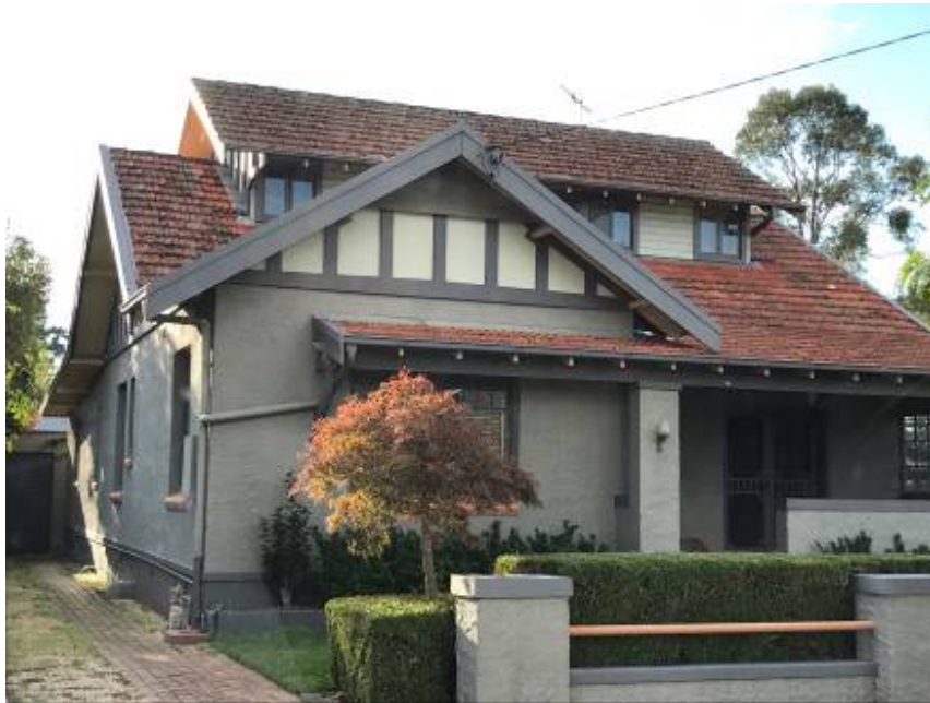
Gable roof features – 2 nd storey additions – Multiple roof forms
