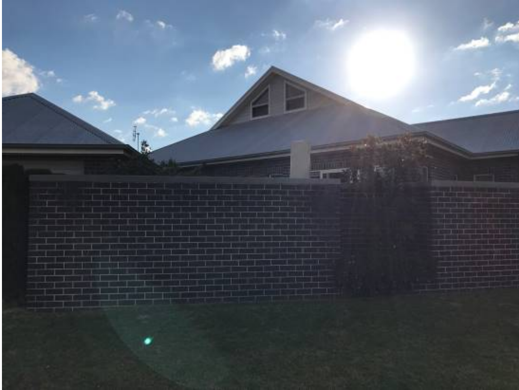
Corner of Williams Close and Melrose Street – Gable windows - not even traditional style but modern angular – colorbond fascia – colorbond gutters – contemporary dark brickwork
