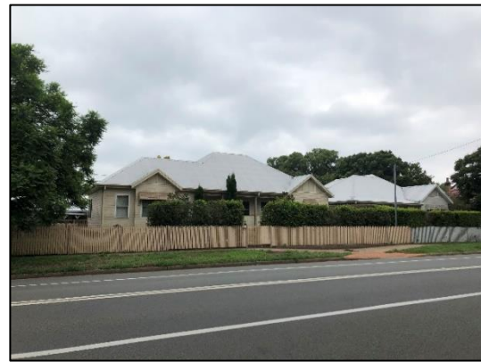
Photo 8: View from Belmore Road looking at existing development opposite the site.
