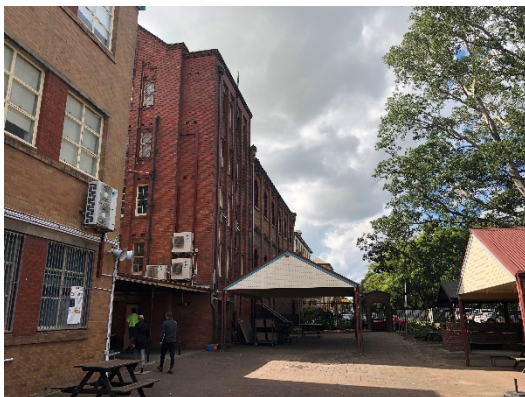
Courtyard south of Block G view east
