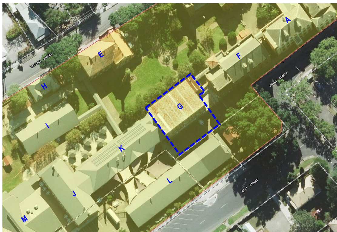
Figure 3: Aerial view. Block G and outdoor area outlined in blue (Source: LPI SIX Maps viewer)
