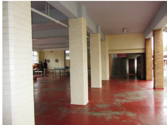
Plate 7: The existing open undercroft area. (JCHD 6931)
