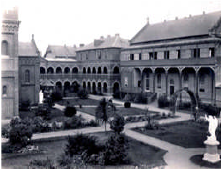
Plate 4: Block F building with bullnose verandah. (St Marys HS)
