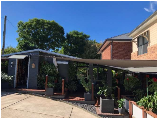
Photo 15 view from the backyard of 26 Catherine Street (supplied by Council).
