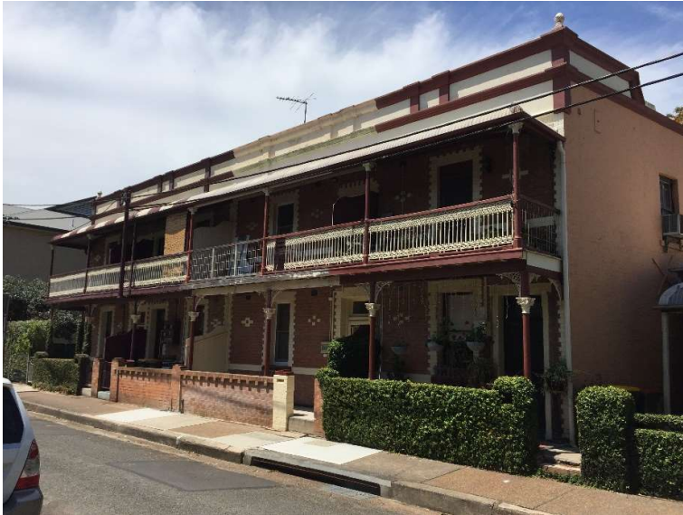
Photo 7 Street Frontage of Fry's Terrace (15-21 Catherine Street) (2020)
