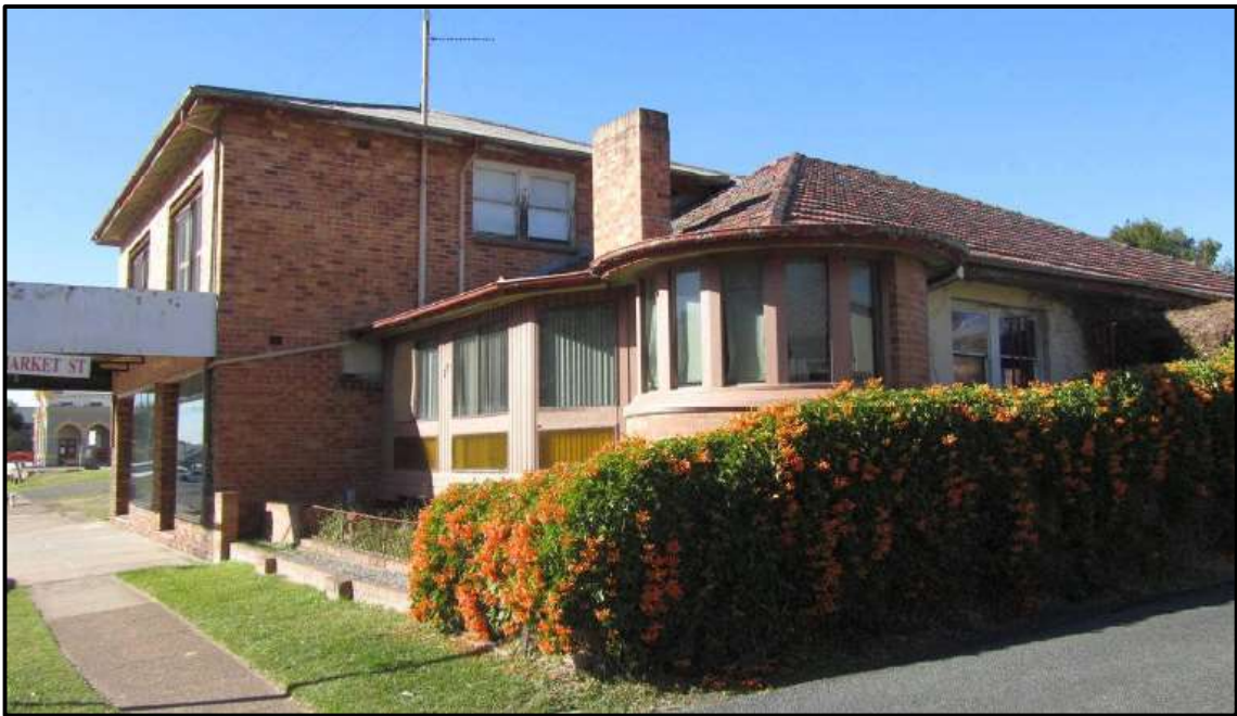
Photo 3 - Shop and residence viewed from the corner of Swan & Market Streets (Source: JCHD, 2021)
