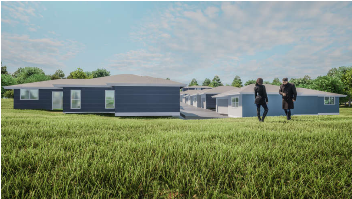
Figure 4: Rear view: This image shows the central driveway to the rear and the typical aesthetic of the proposed single storey units. Once again, a simple Hamptons style is utilised to create an appealing and lasting aesthetic for the development
