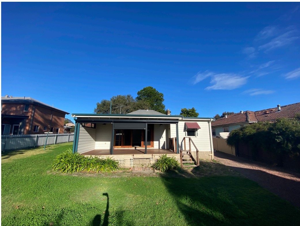
Figure 7: Rear Facade of 144 Lawes Street East Maitland (Source: Hoover Group)
