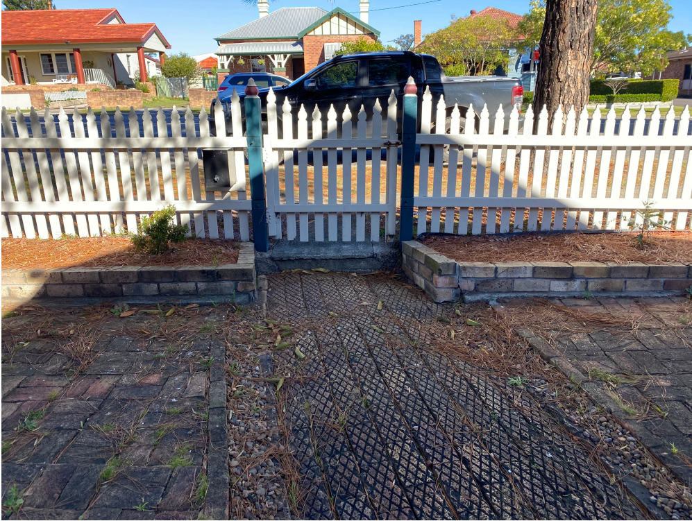
Source 14: Existing Front Entrance Step (Source: Hoover Group)
