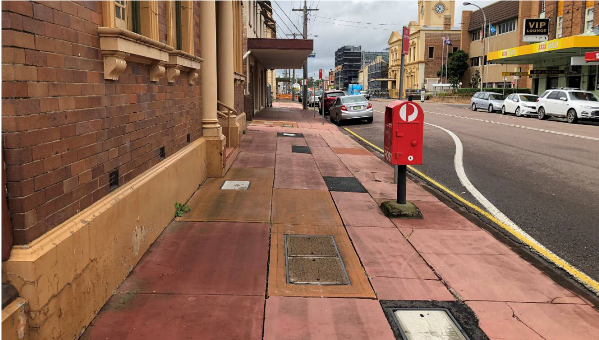
Photograph 7 – Footpath along High Street frontage
