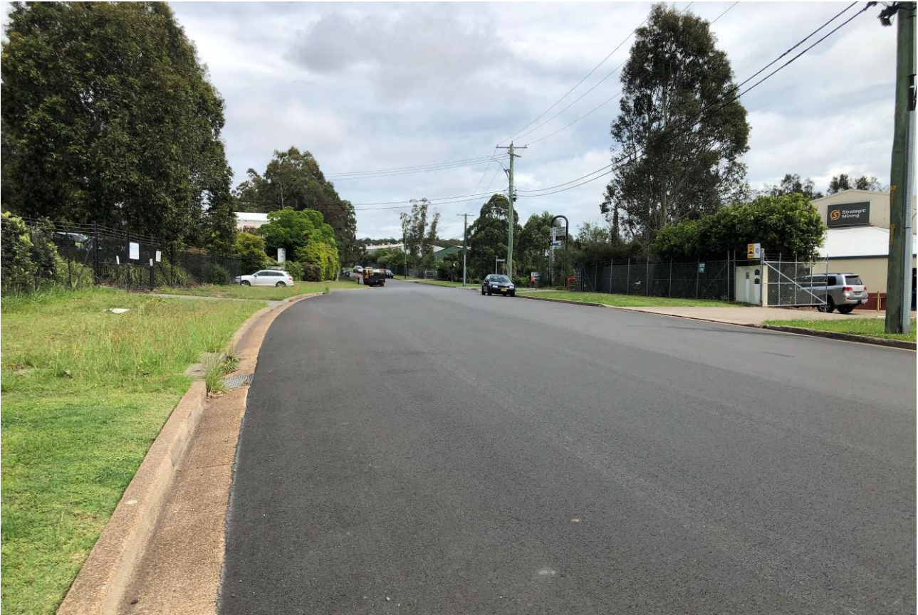
Photograph 4 – Huntingdale Drive in the vicinity of the site.
