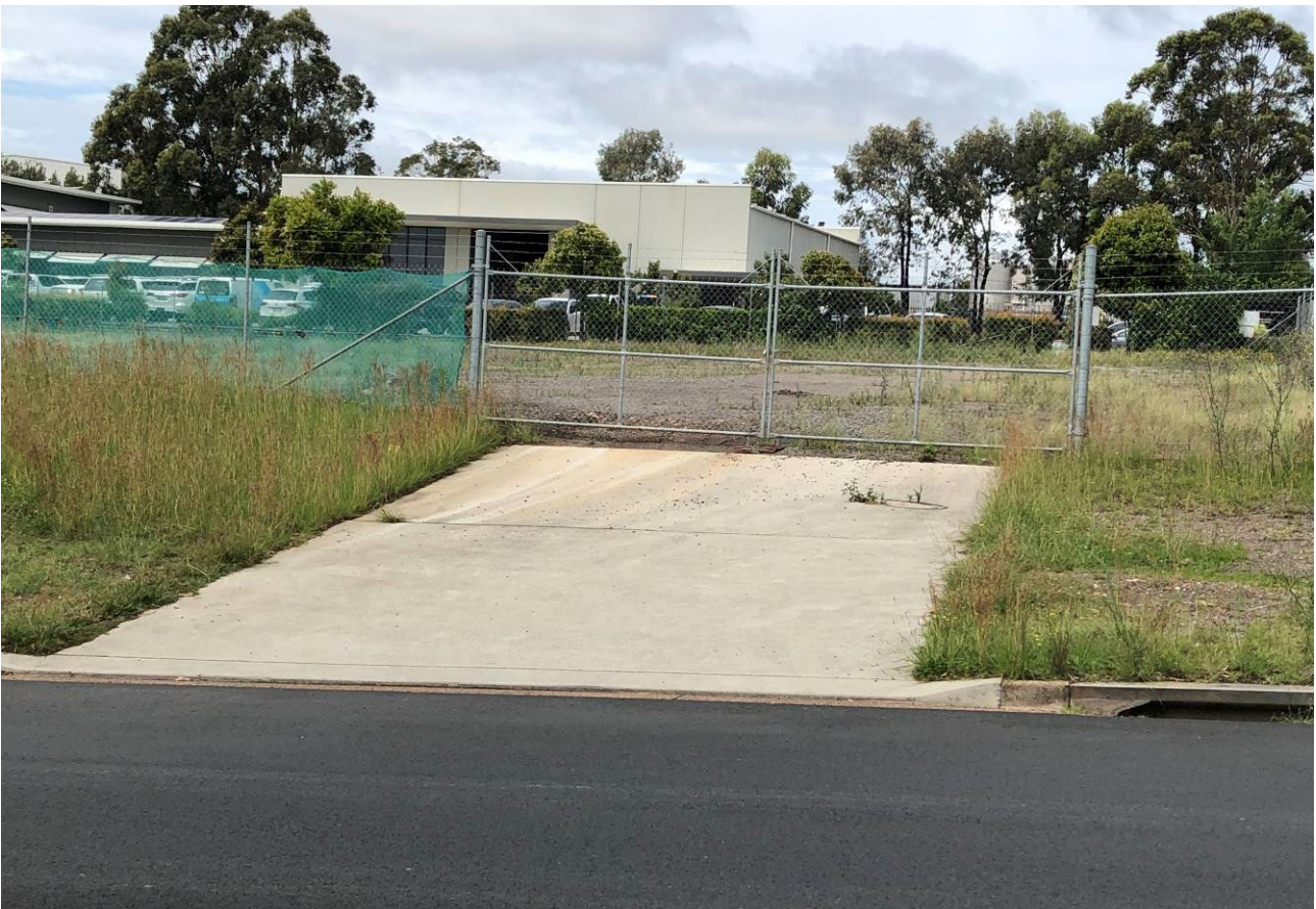
Photograph 2 – Existing site access
