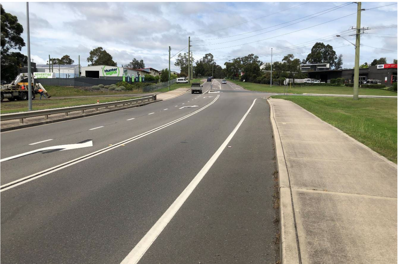
Photograph 5 – Thornton Road / Huntingdale Drive intersection.
