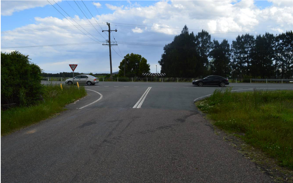
Photograph 7 – Raymond Terrace Road / Martins Wharf Road intersection
