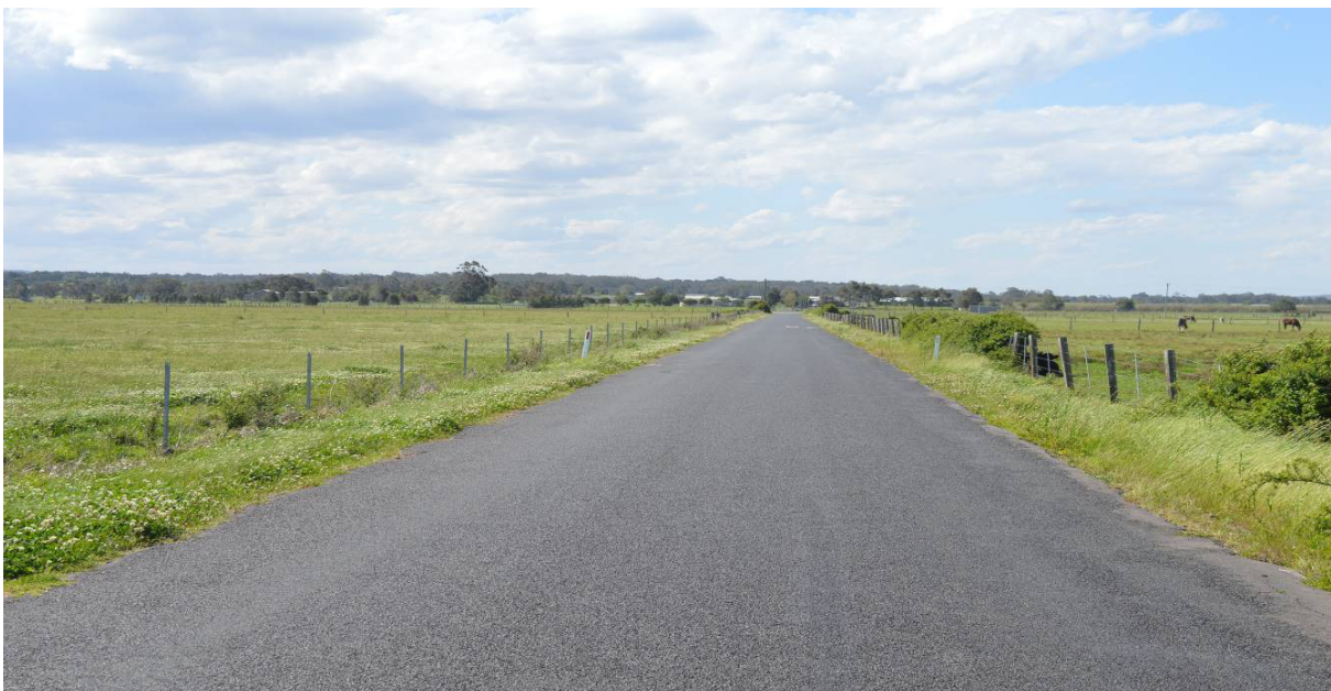
Photograph 5 – Martins Wharf Road adjacent to the site
