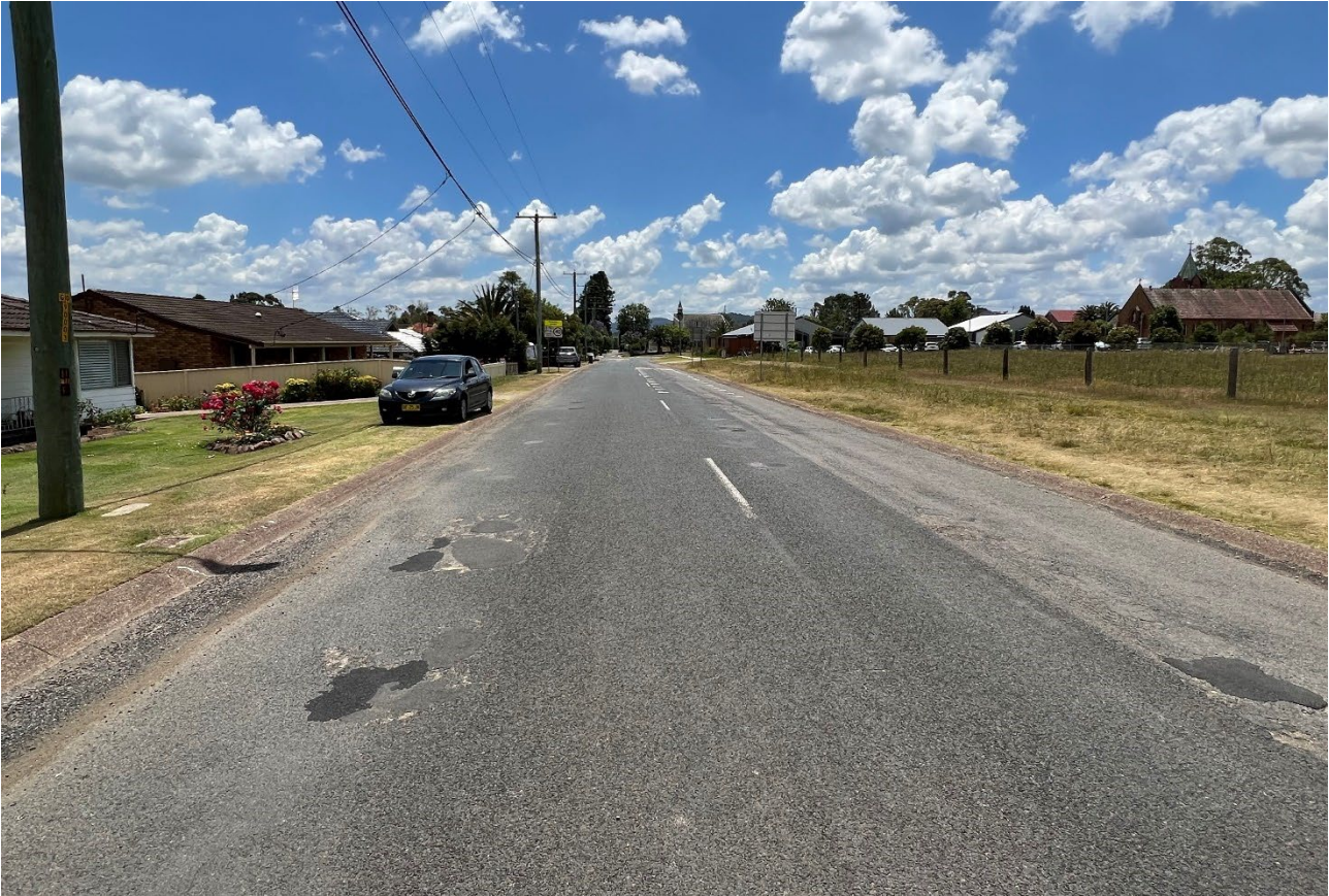
Photograph 4 – Station Lane near New England Highway.
