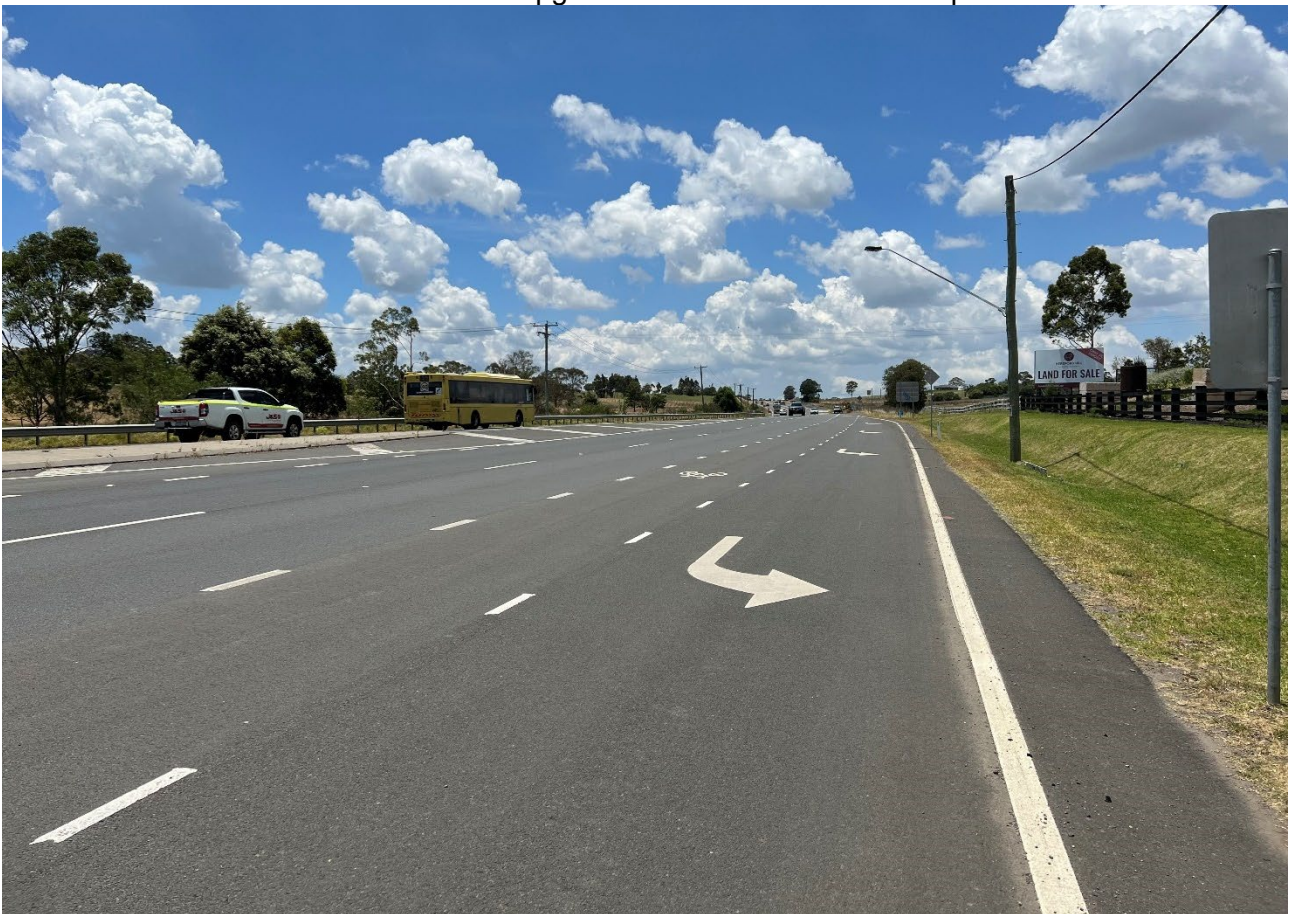
Photograph 3 – New England Highway near Springfield Drive.
