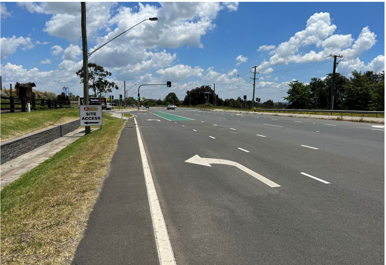
Photograph 2 – New England Highway / Springfield Drive signalised intersection.
