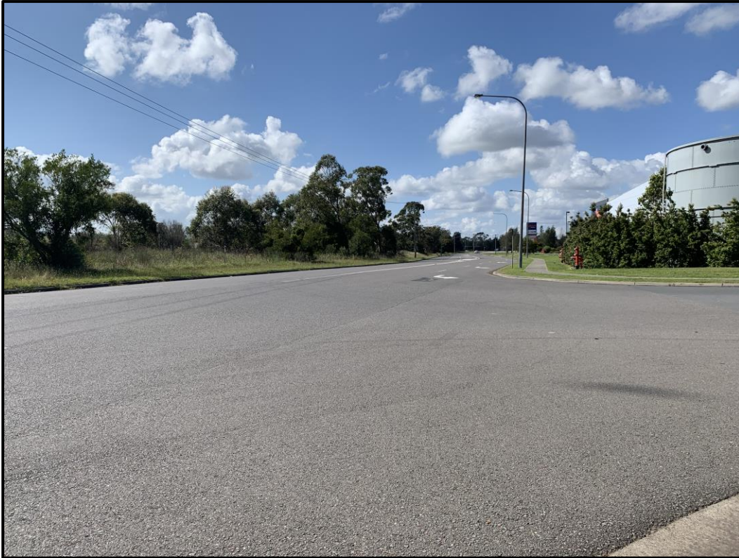
Photo 3 –Anambah Road with Mustang Drive to right of photo showing intersection layout looking south
