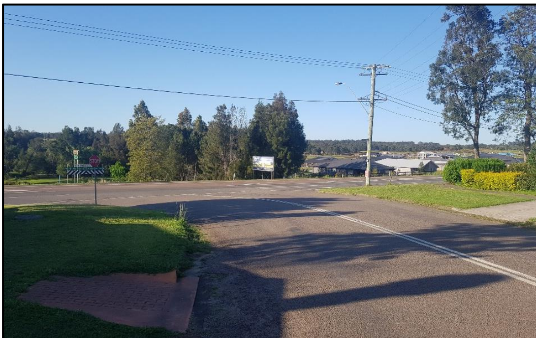
Photo 1 – Windermere Road on approach to the New England Highway.
