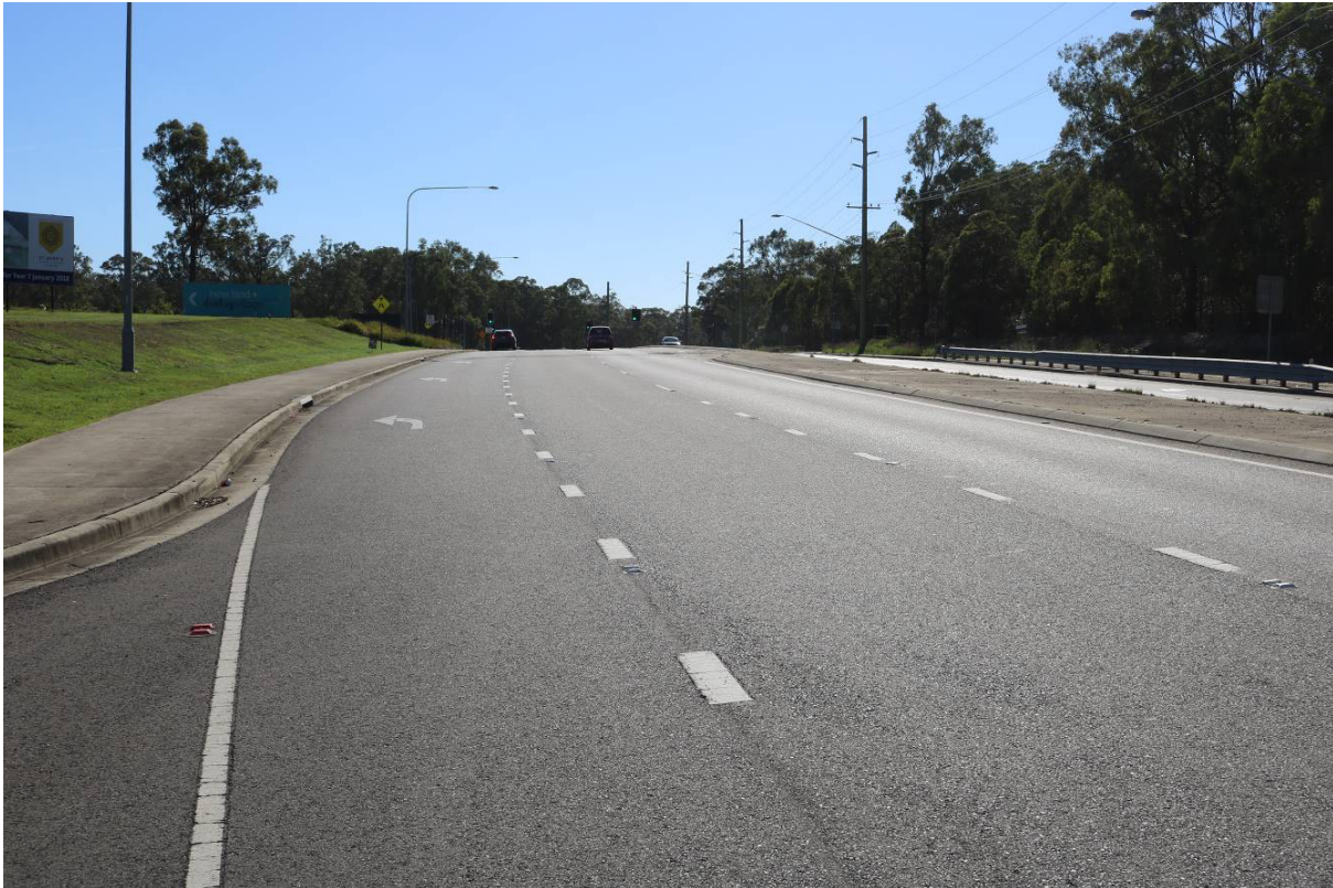
Photograph 2 – Raymond Terrace Road at Settler’s Boulevard intersection
