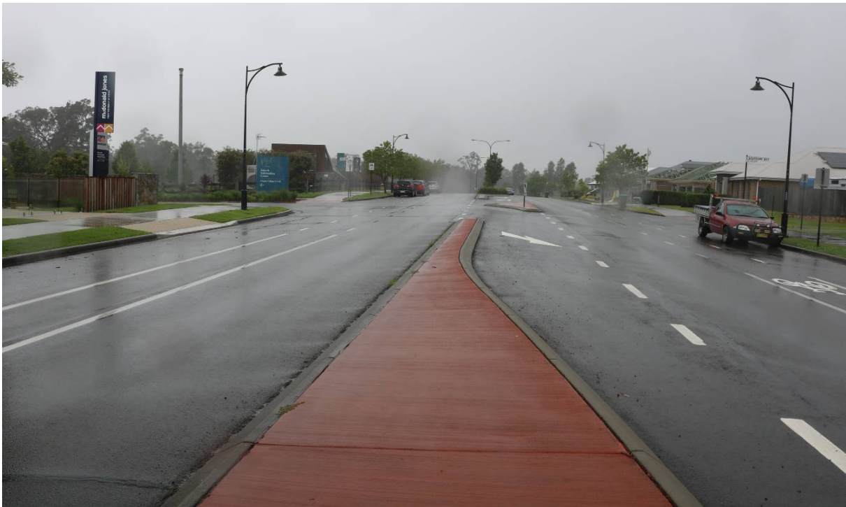
Photograph 5 – Settler's Boulevard at Cora Way intersection
