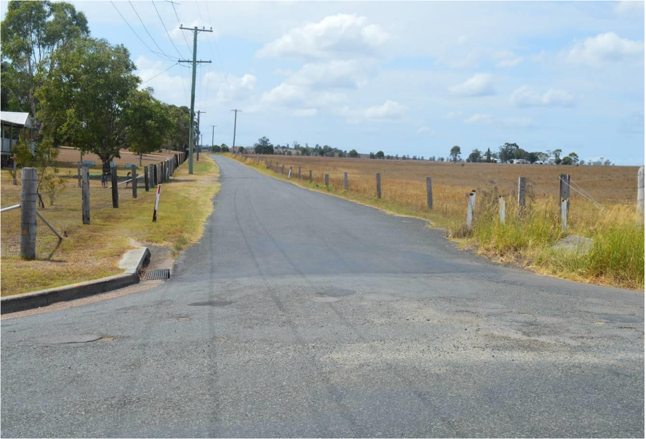
Photograph 5 – Christopher Road at Station Lane
