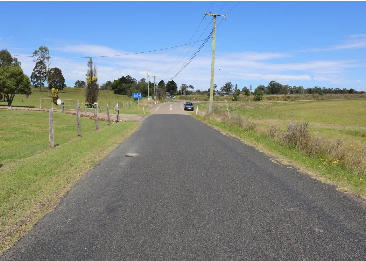
Photograph 4 – Station Lane near the site
