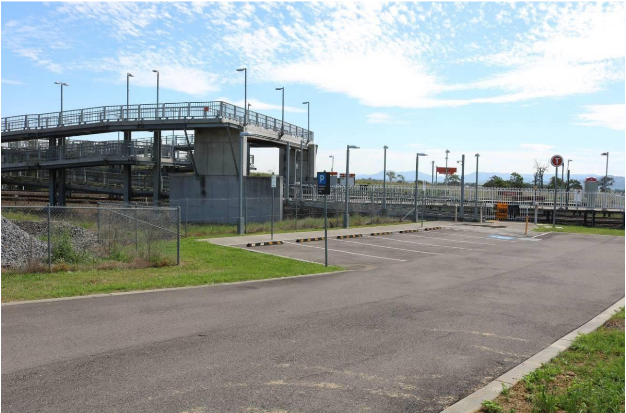
Photograph 9 – Lochinvar Train Station
