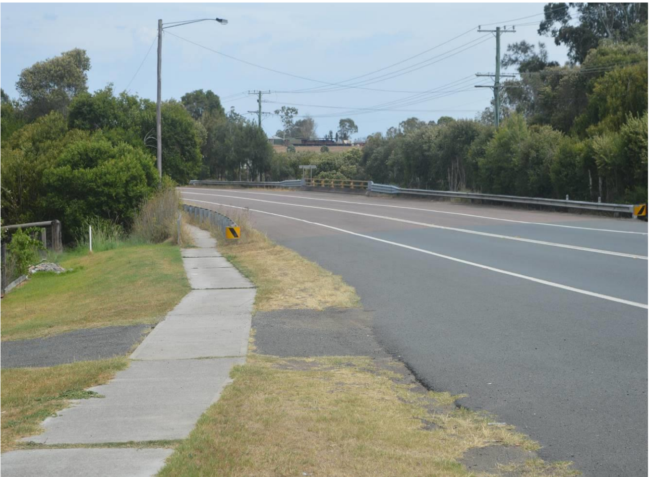
Photograph 3 – New England Highway near Station Lane
