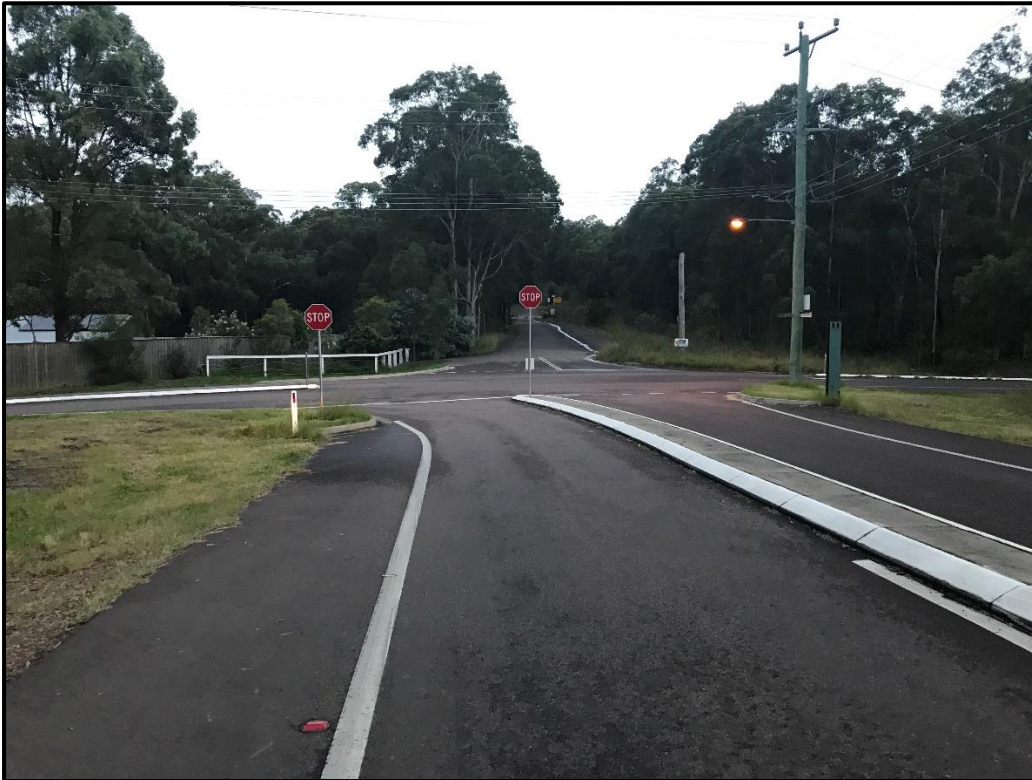
Photo 1 – Louth Park Road approach to Mount Vincent Road
