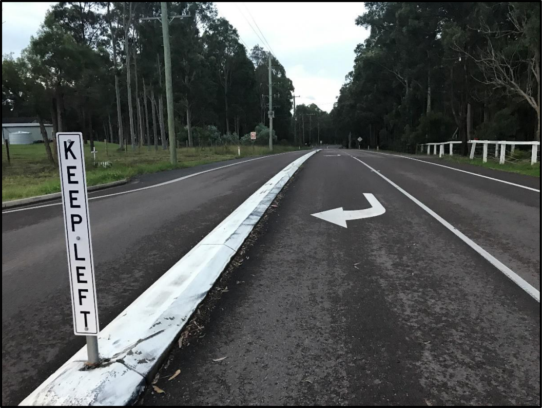
Photo 4 – Right turn lane on Mount Vincent Road for traffic turning into Louth Park Road
