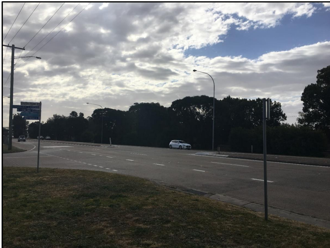
Photo 1 – Intersection of New England Highway and Louth Park Road
