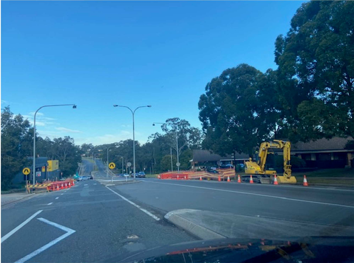
Figure 4: View from Stronach Avenue looking south towards the site
